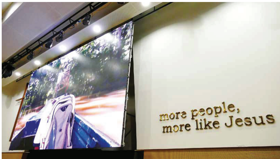
The Aoto MXC4 LED wall was aligned with the existing features
