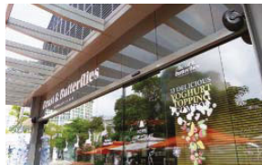
The outdoor seating and ninth level pool areas are catered for by EV Evid 4.2T dual 4-inch weatherproof speakers
