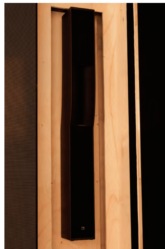
Concealed within door frames, L-Acoustics Syva columns provide horizontal coverage
