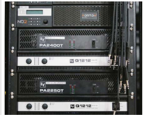
The EV C8.2HC ceiling speakers are powered by EV PA2250T and PA2400T amplifiers
