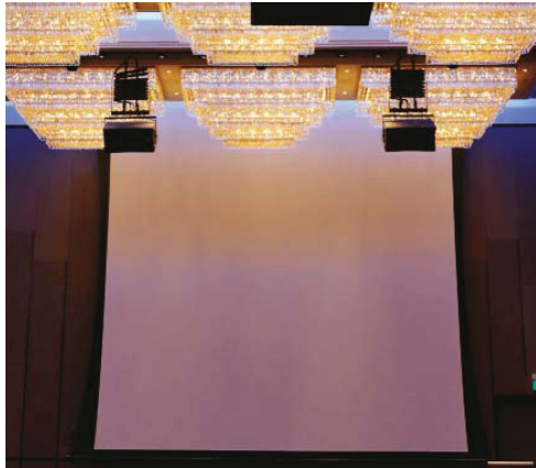
A main LAV Hariz BN 4m x 6m screen receives its display from a Panasonic PT-RZ970 8,000 ANS-lumens laser projector
