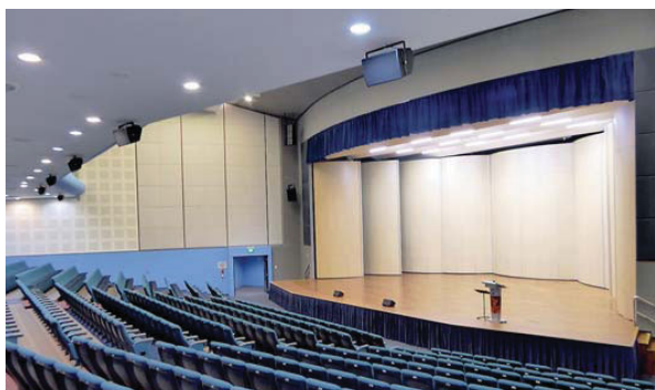
The under balcony seats are now covered by six NF8 loudspeakers
