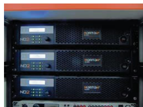
Three ND2 amplifiers power the L-R i1212W and six NF8 under balcony speakers
