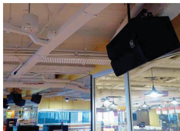
Four EV TX1152 speakers are powered by dual Q1212 amplifiers
