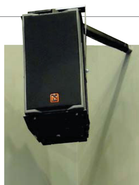
One of the L-R i1212W speakers affixed to reinforced concrete beyond the fire rated wall
