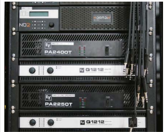
The EV C8.2HC ceiling speakers are powered by EV PA2250T and PA2400T amplifiers
