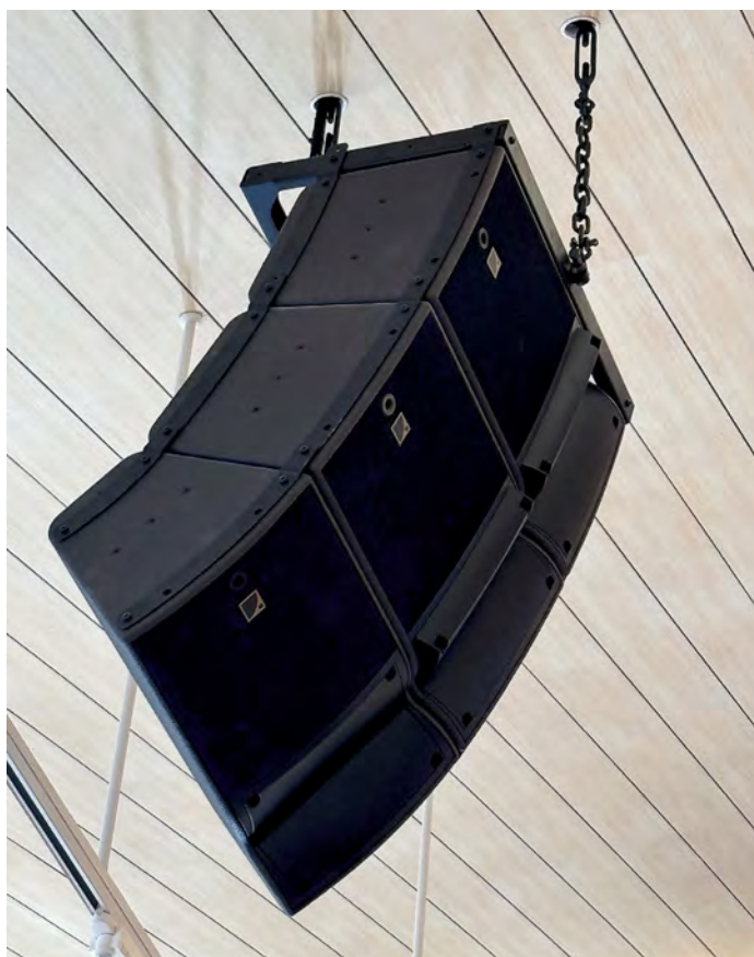
Each L-R array comprises two A10i Focus and a single A10i Wide cabinet
