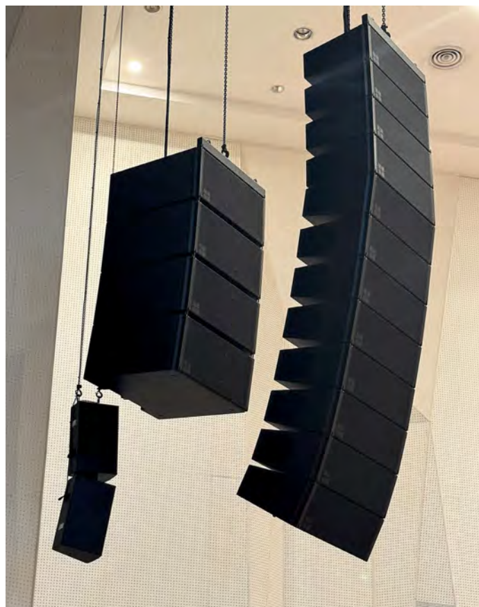
Suspended L-R pairs of KSLi and KSLi-Subs provide consistent coverage
