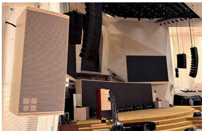
Wall-mounted Y17P enclosures serve as powerful side fills
