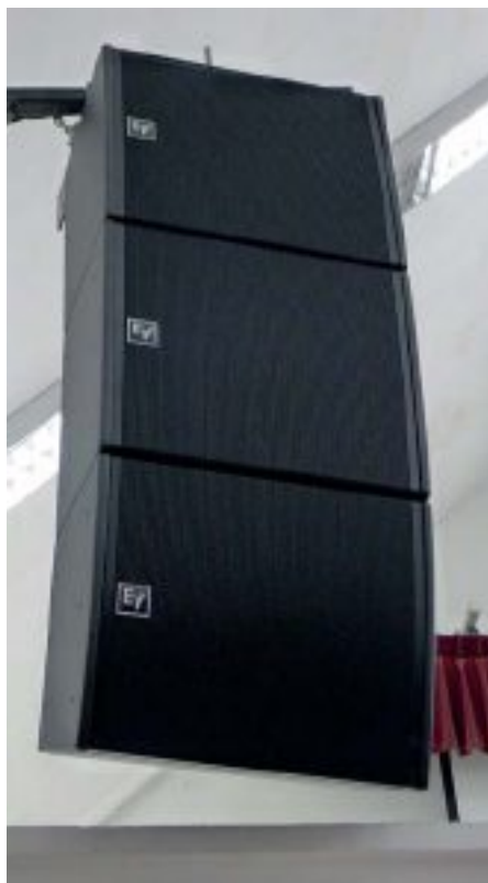
Each EVA2082S hang weighs 108kg including the bracket
