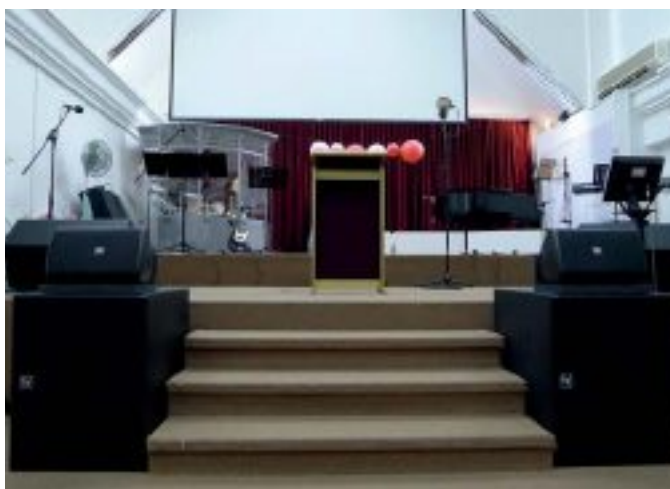
Dual floor standing EVA2151S subwoofers with ZX1i cabinets providing front fills
