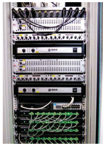
(L to R): Racked analogue equipment for the EV ELX112 portable stage monitoring; Panasonic PT-EZ720 and PT-EZ570 LCD projectors, Samsung screens and EV ZX190 8-inch enhance the meeting rooms; The meeting rooms in Block 14 are each equipped with Crestron DMPS-300-C and DMPS-200-C systems for A/V presentation control
