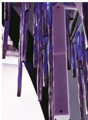
The Ballroom's FOH system combines L-R wall mounted dual Coda Audio CoRay4i line source column speakers with SC18 dual 18-inch subwoofers
